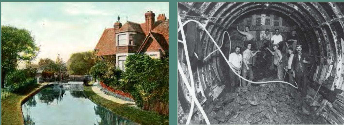
Before the estate - New River (left). Tunneling and building Manor House Tube (right).
